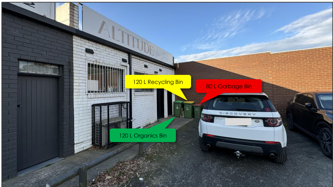
Figure 4 2452 Warburton Highway Waste Bin Storage Area (Salon)
